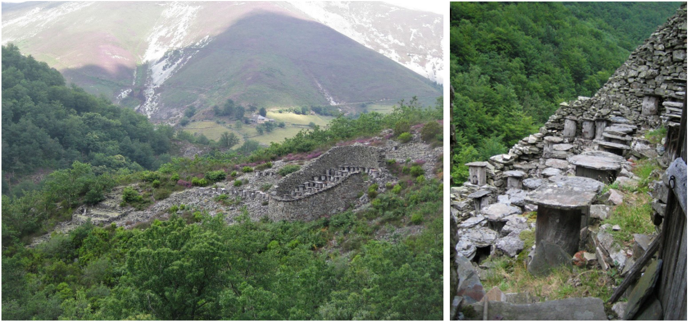
Fig. 3. Examples of stone structures built to protect apiaries from bears in the Cantabrian Mountains (Photos: FAPAS).
