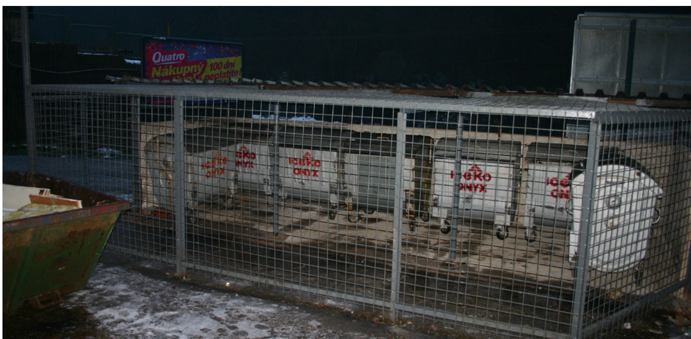
Fig. 7. Metal cage constructed to prevent bears gaining access to standard refuse containers (Photo: Robin Rigg).
