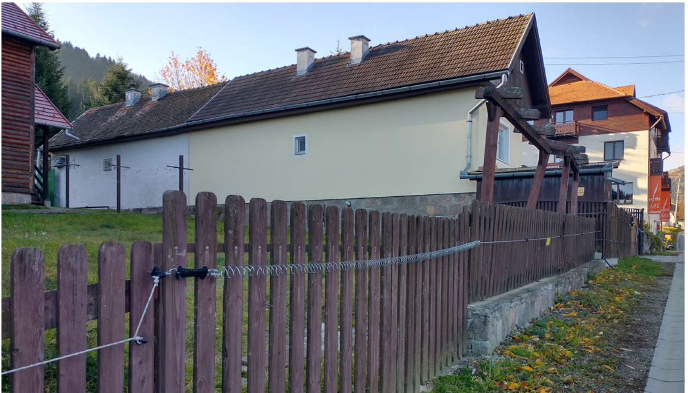
Fig. 8. Single electrified wire mounted on an existing wooden fence to deter bears from entering a garden (Photo: Robin Rigg).
