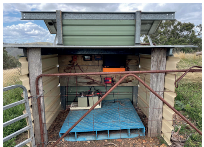
Fig. 7. Solar powered energiser in a paddock at Box Hill sheep farm (Photo: Jodie Healey).
