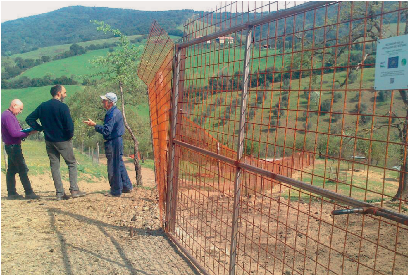
Checking use and status of installed fences.
