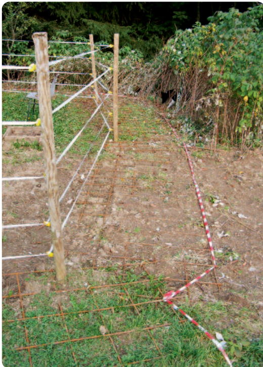
Photo 12 - Electric welded mesh to prevent digging, tried out experimentally at the base of electric fences (E. Bonapace, APT Forestry and Wildlife Dept. Archives)
